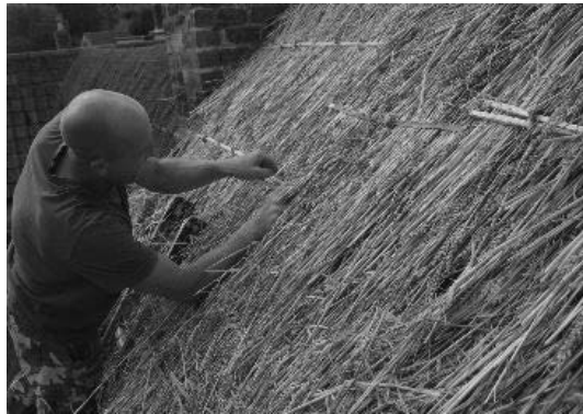
1: Ickleton: long straw being secured by local master thatcher, Mark Treadwell.
