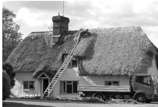
2: Rickling Green – work in progress
